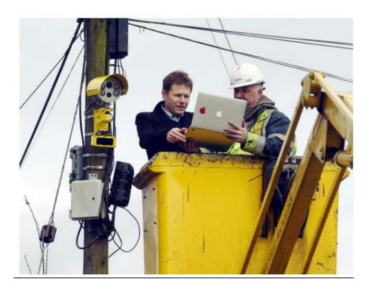
The Safe-Speed ANPR camera is a mains powered unit which is usually fixed to a pole above the road and requires authorisation from the utility company to connect to the supply. It is not intended to be moved from site to site.
